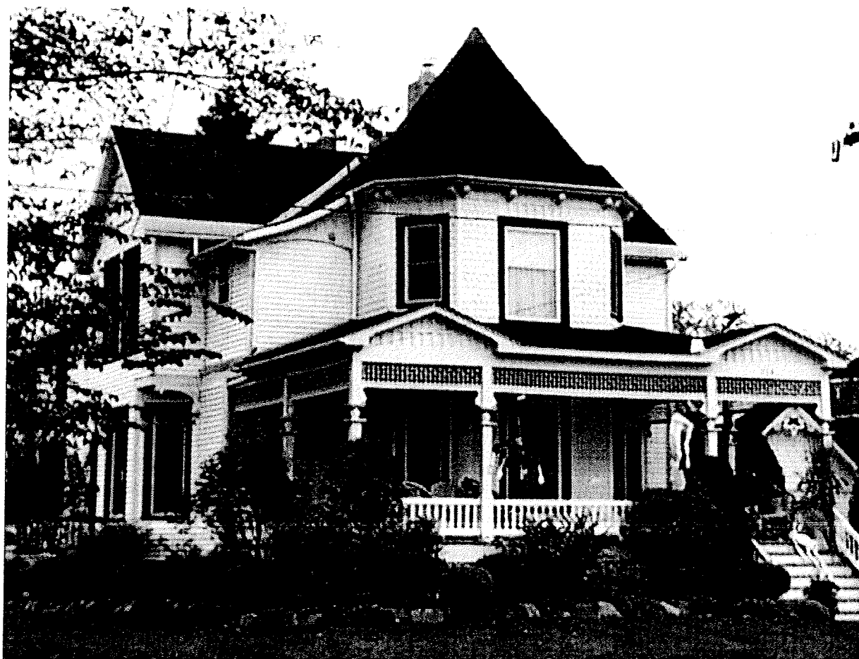
Photograph – Condition of building in 2006
